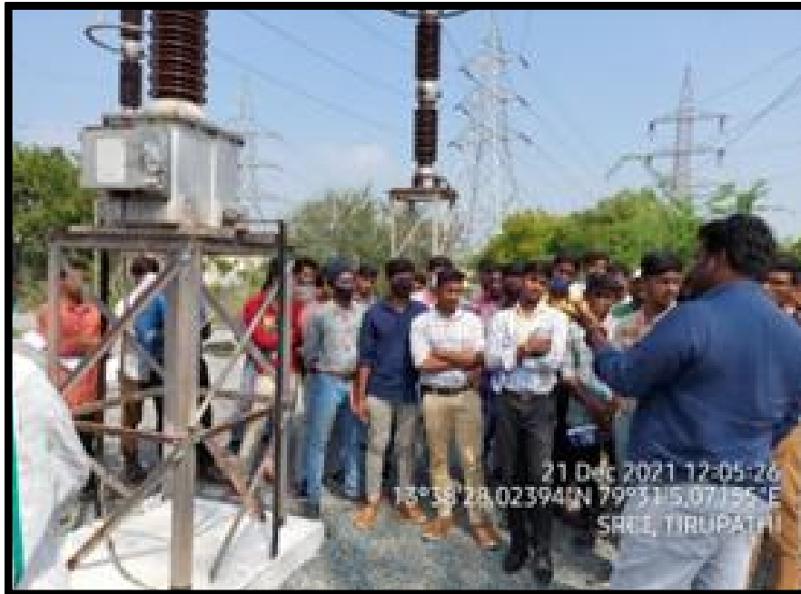
A field visit to 220 kV Substation, Renigunta
