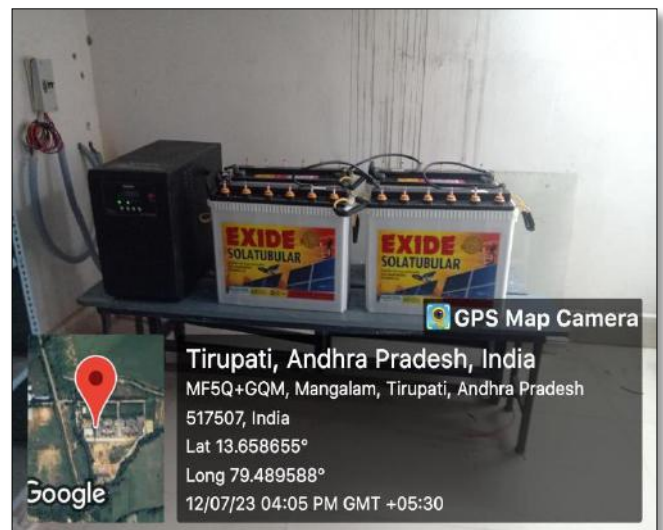
Battery and Inverter Setup
