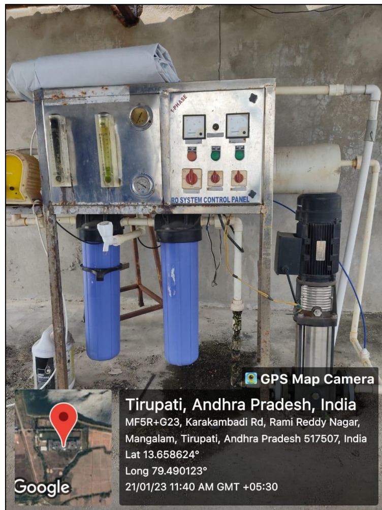
Reverse Osmosis (RO) System (500 Litres per Hour Capacity) at 3 rd floor (Terrace)
