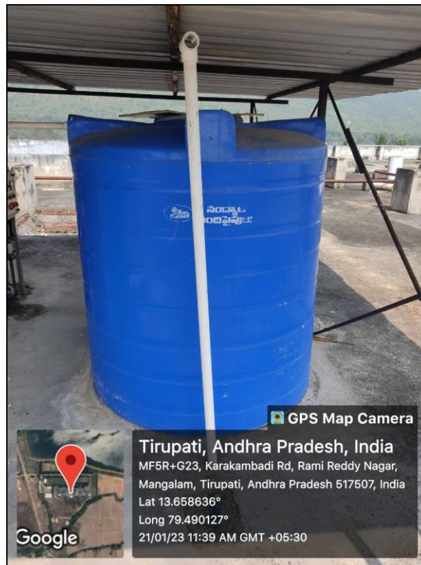
Water Tank at Engineering Main Block with Capacity:2000 Litres
