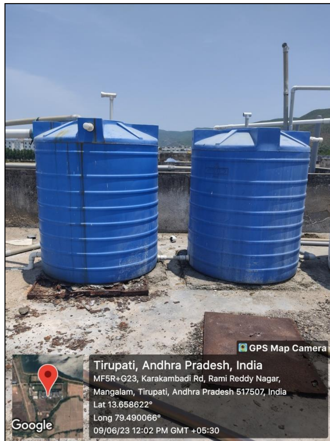
Water Tank (Third Floor) at Engineering Block of with Capacity:1000Litres each (2*1000 Litres=2000 Litres)
