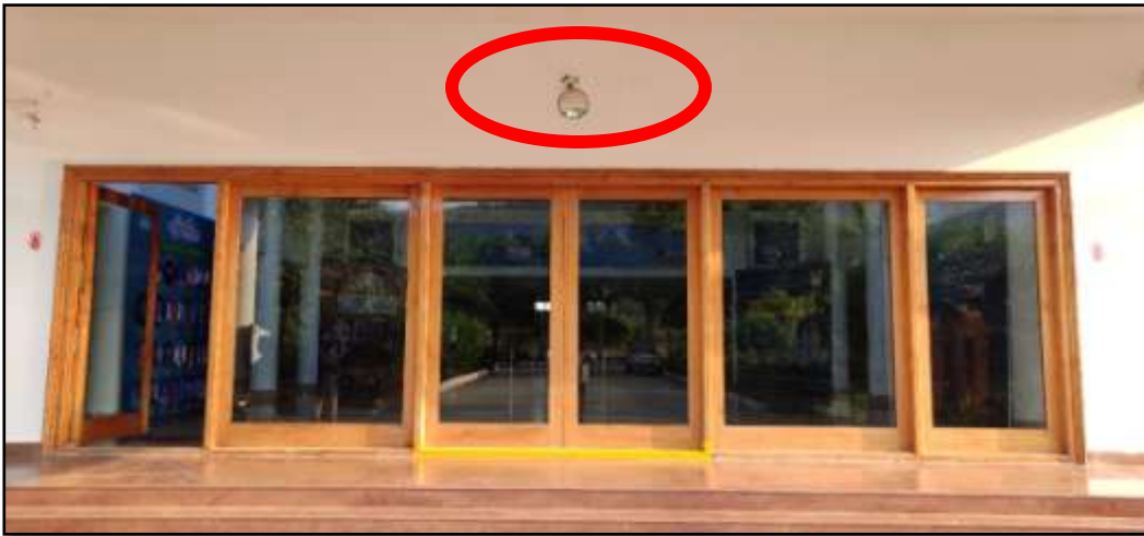
CC Cameras installed at the entrance of the College
